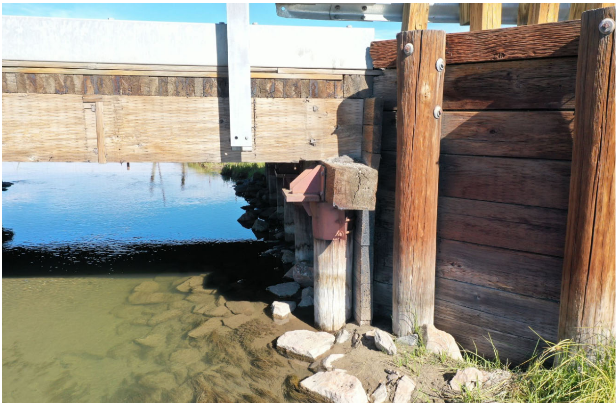
Picture 3 – Abutment and Wingwall
