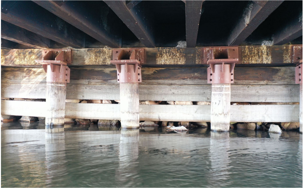
Picture 2 – Girders, Abutment Backing and Piles
